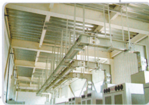
母线设计简单清晰,火灾荷载低 Busway planning is easy, low fire load
